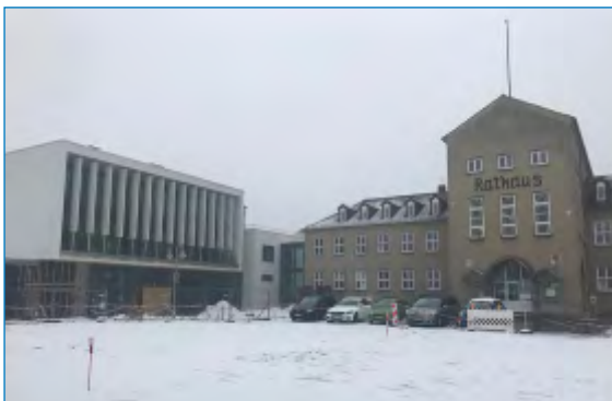
Town hall, Hohen Neuendorf
